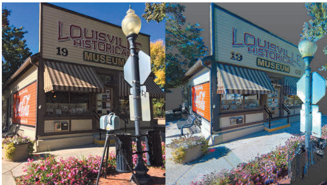
Figure 3: TX6 colored point cloud of building exterior.
