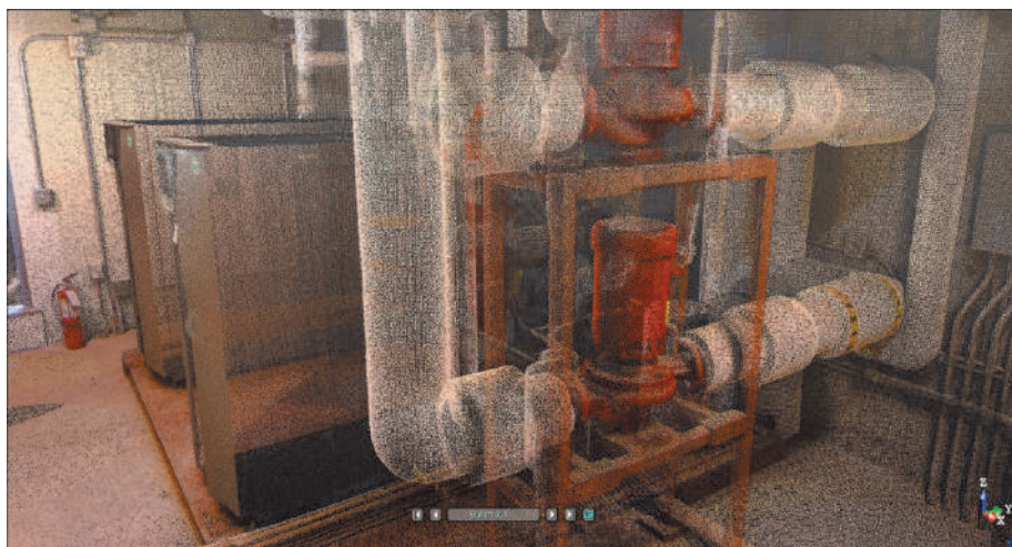
Figure 5: TX6 colored point cloud of building mechanical room.
